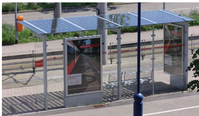
Fig. 3 Solar bus stop in Freiburg in Germany [4]
